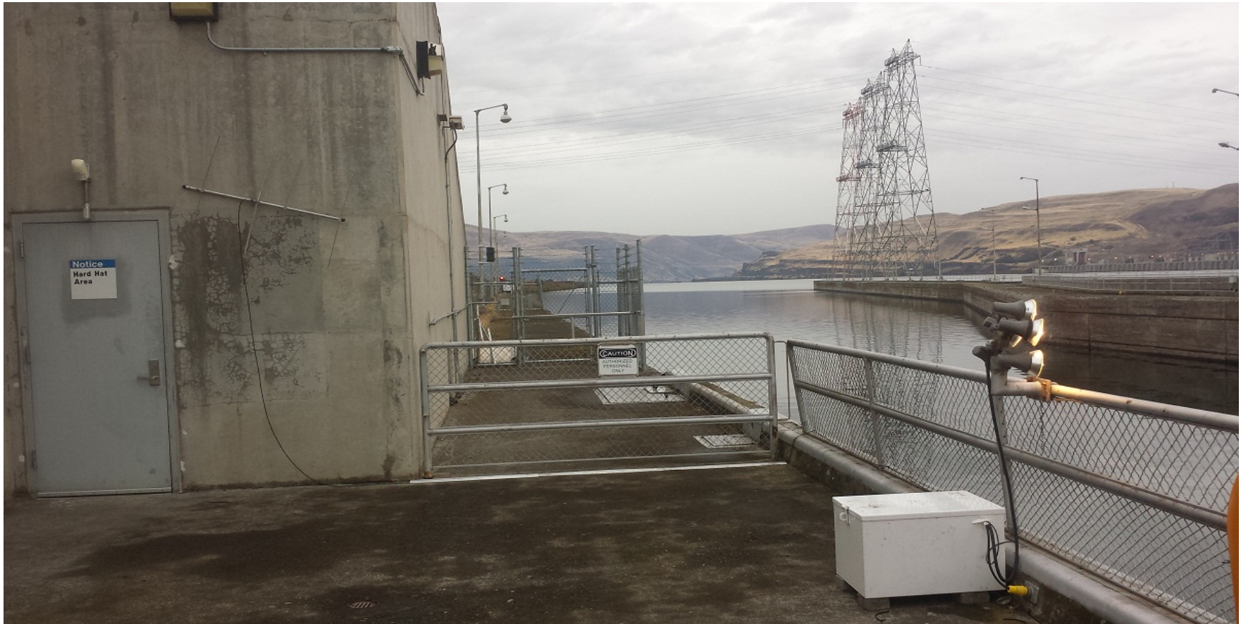
U of I new aerial antenna downstream of the navlock to monitor winter steelhead.
